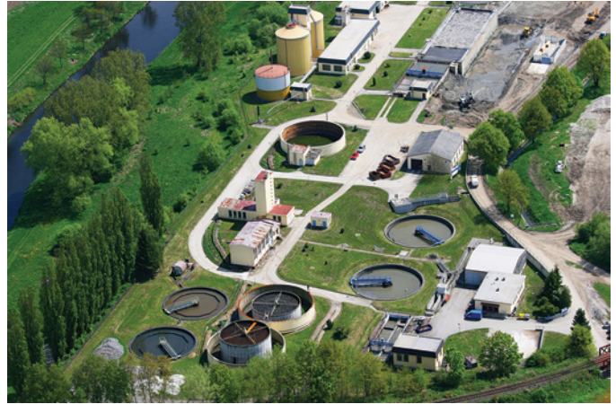
FIGURE 14.8 A wastewater treatment facility.
